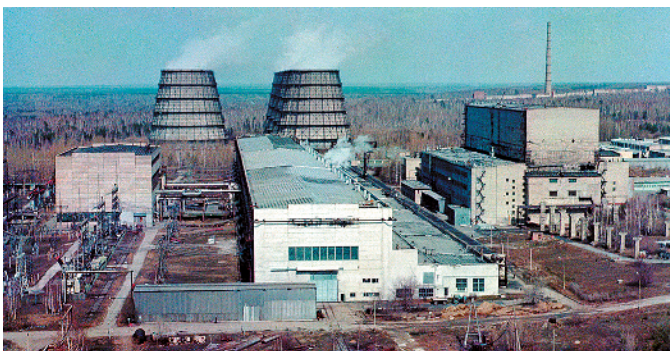
Coal Comfort. This Soviet era weapons-grade plutonium-producing nuclear power facility in Seversk, Russia will be replaced, under NNSA leadership, with a coal burning facility.
